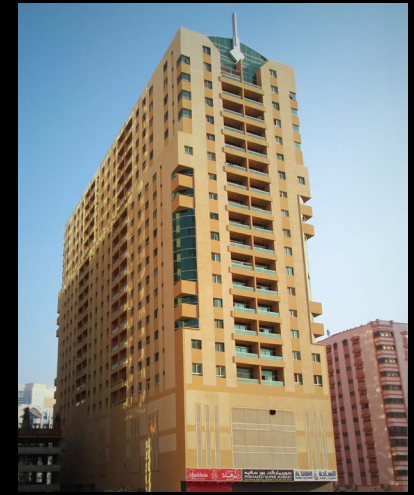
AL MIDAN TOWER
