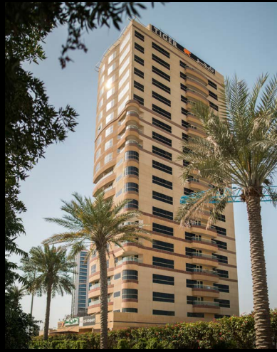
AL DANA TOWER
